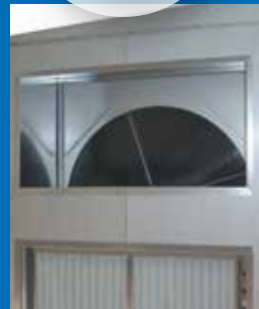
Rotary heat exchanger
