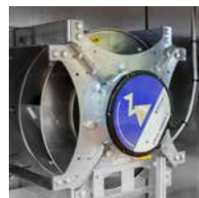
Plug fan with electronically commutated motor
