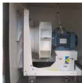
Plug fan with induction motor
